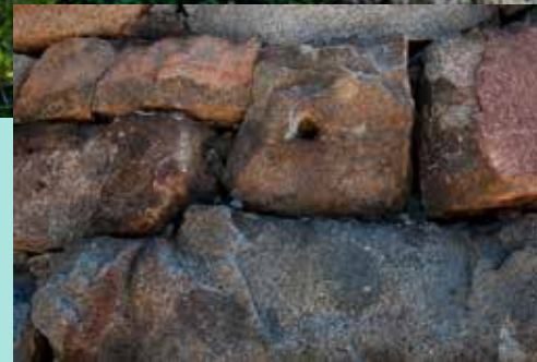
Above: China Wall, constructed by Chinese railroad workers. The stones fit perfectly with no mortar.
