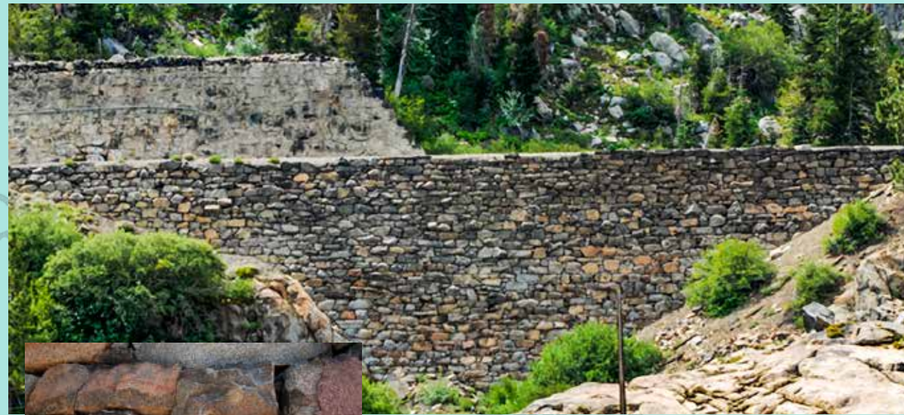
Above: China Wall, constructed by Chinese railroad workers. The stones fit perfectly with no mortar.
