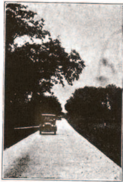
Concrete Pavement on Lincoln Highway, Allen County, Indiana
