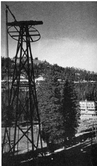
One of the 13 towers of Sugar Bowl's ultra-modern chair lift, which will take you 3200 feet (1000-foot rise) in six minutes.
