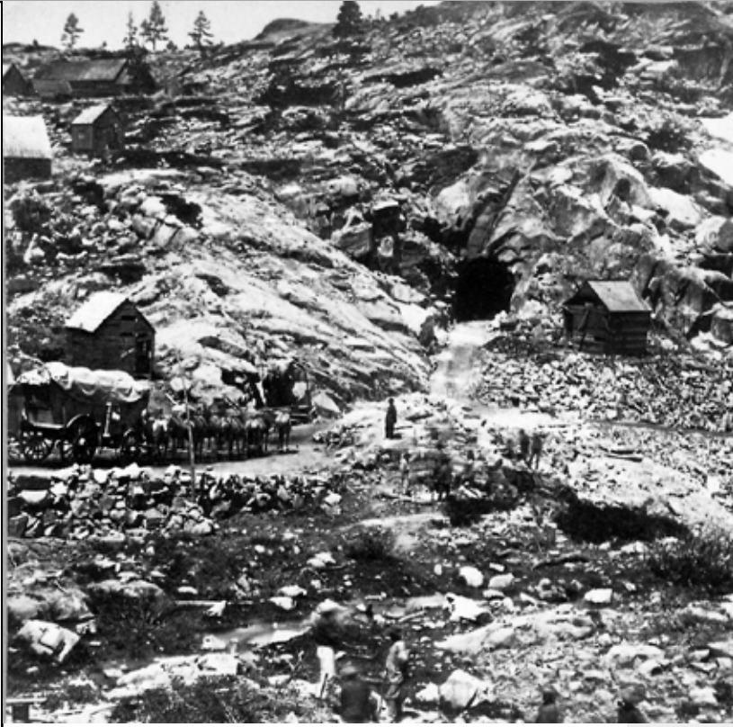
Alfred A. Hart. East Portal of Summit Tunnel #199 and wagon road from Tunnel 7; 1/2 of a stereopticon slide
