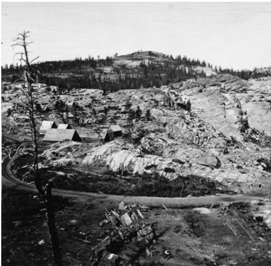
Alfred A. Hart, titled, "Camp Summit Tunnel, Mt. King in the distance" It looks like Donner Ski Ranch was Mt. King. In the foreground is the Donner Lake Dutch Flat Wagon Rd., essentially the route of the Lincoln Highway.
