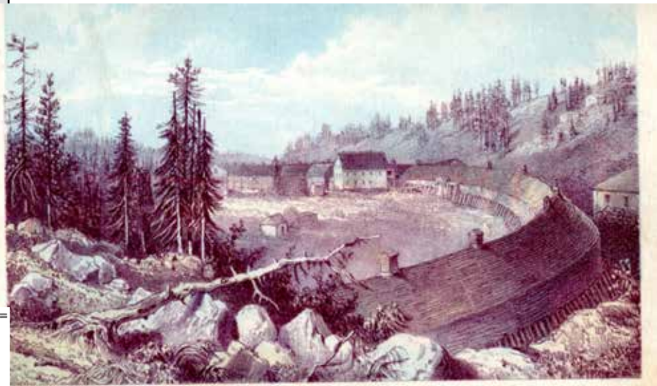
SUMMIT STATION AND EXTERIOR OF SNOW SHEDS.
