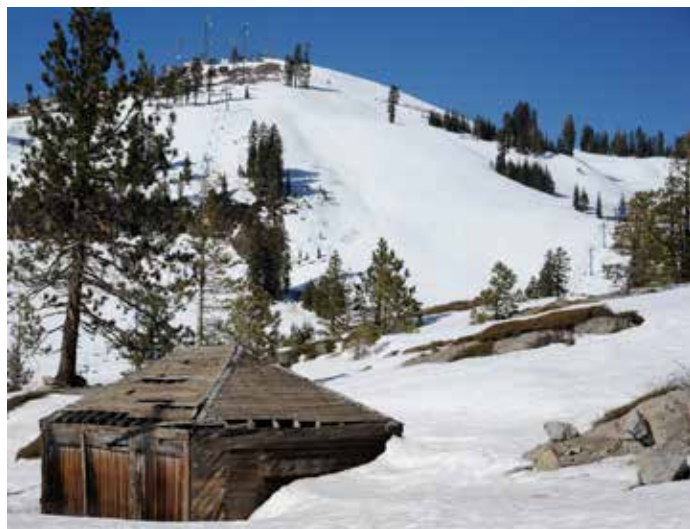
Old garage that could really use restoration. The building sits on Old 40 just down from the summit. It was the garage for the weather station - see the next page. It is leased by Norm Saylor from the UPRR
