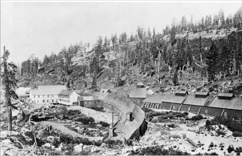
Photograph of Summit Hotel I. The curved snowshed leads to Tunnel 6. The other wing includes the roundhouse (with the small cupola) for turning engines around.
