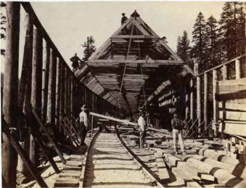
246. Constructing Snow Cover. Scene near the Summit.
