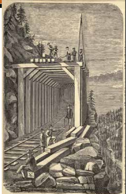
163. Frame for Snow Covering, interior view.
