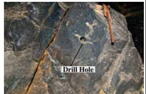
Tool marks still on the walls of Tunnel 6.
