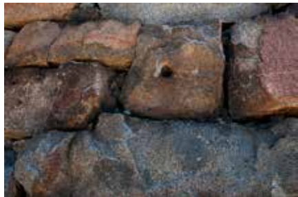
Above, China Wall. The rocks are held together by nothing but their weight and accurate placement. Look closely for tool marks like the drill hole to the left and the marks above which come from splitting the rocks. The rocks in China Wall came from the tunnels.
