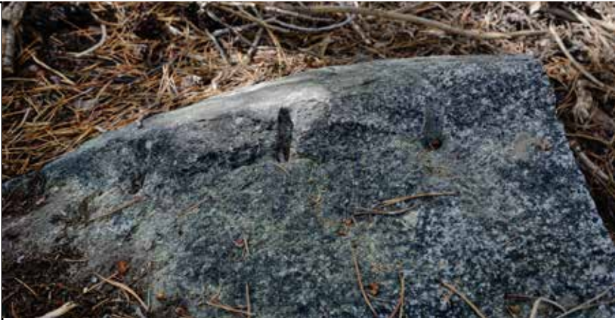
Granite rock with wedge holes. Workers drilled a line of small holes in the granite and then inserted wedges. The wedges were hit in succession until the rock split. You can see many of these rock splitting artifacts in China Wall stones.
