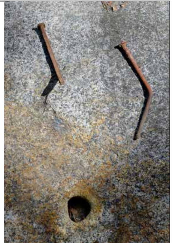
Square nails (left on site) and an old drill hole in granite.
