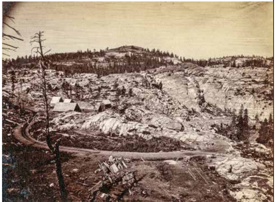
Alfred A. Hart #116 "Camp Near Summit Tunnel" showing buildings in the Chinese work camp called "Summit Camp." The road in the foreground is the Dutch Flat Wagon Rd. which would mostly become the Lincoln Highway in 1913
