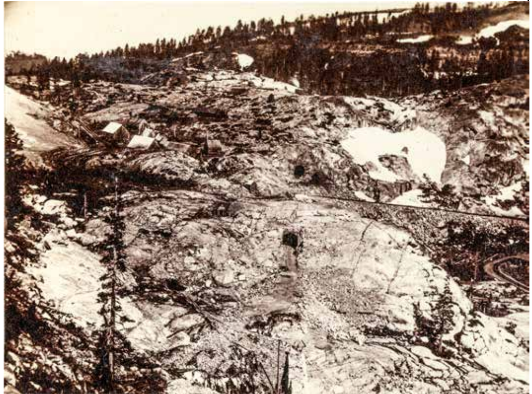
Alfred A. Hart #202 "East Portals of Tunnels No. 6 and 7 from Tunnel no. 8" showing buildings in the Chinese work camp called "Summit Camp." Wendell Huffman of the Nevada State Railroad Museum in Carson City, says that after analyzing the Alfred A. Hart photographs of Summit Camp that he sees 16 buildings (see sidebar below).
