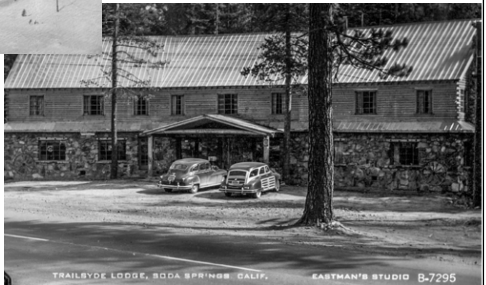
Right, Trailsyde Lodge which used to be at Big Bend.
