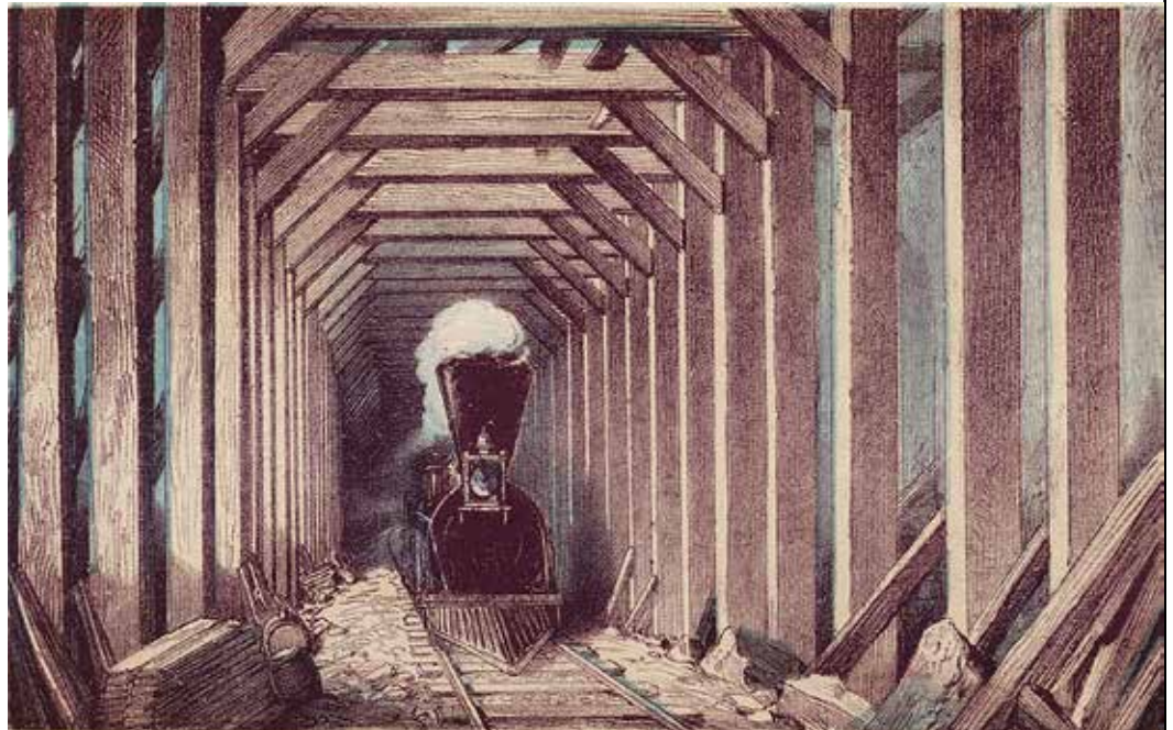
Above: Summit Station and Exterior Snowsheds Below: Interior of snow-sheds
