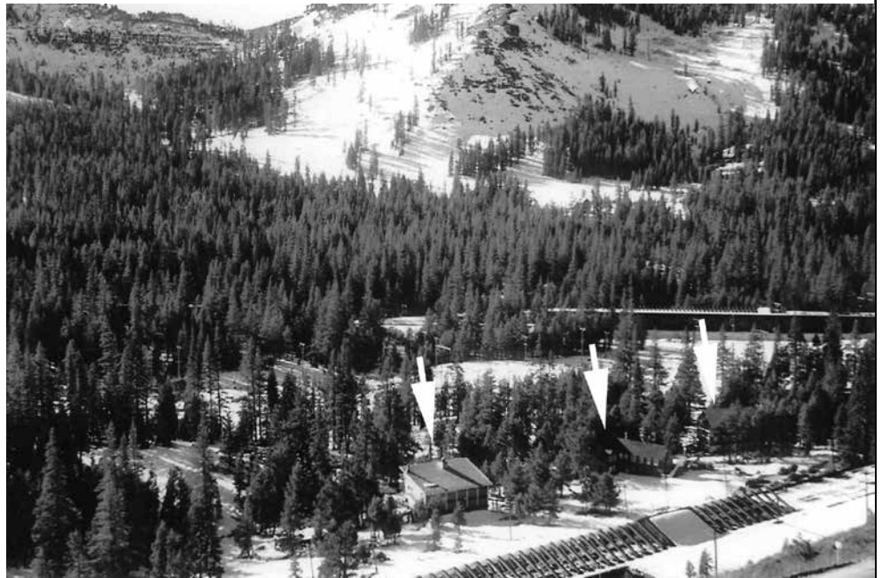
1951 - Three lodges on Old Donner Summit Rd. (the Lincoln Highway dirt road) under the arrows: Oakland, left; Travis (Macintosh), center; and Alpineer, right; along with snowsheds leading to the two tunnels.
