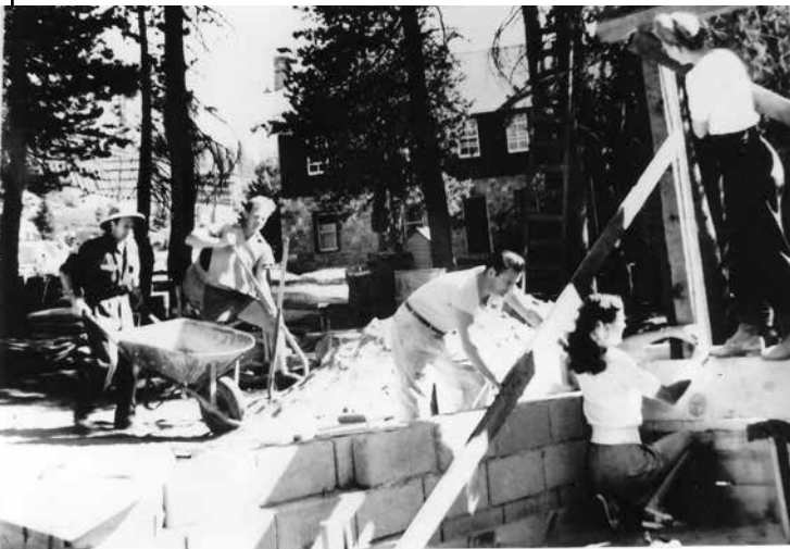
Building the Alpineer Lodge, 1947-48 - Macintosh Lodge in the background.
