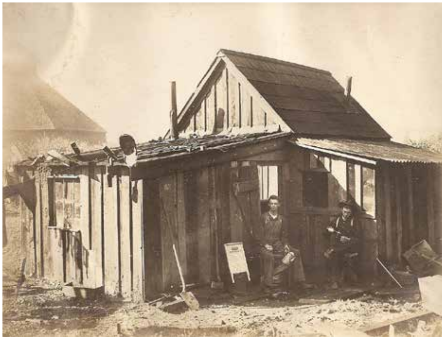
Railroad workers on Donner Summit. To the left is the building housing the turntable which turned around helper locomotives after they'd helped trains up to the summit. Date unknown
