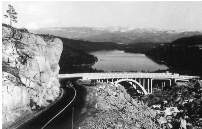
Donner Summit Bridge, 1933. Note the continuous striping. Dashed striping started with WWII to conserve materials.
