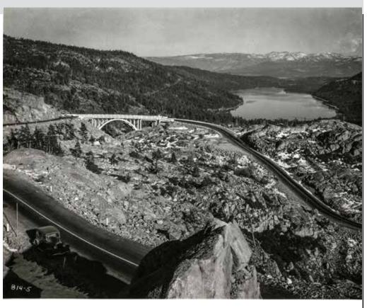
Picture of the Donner Summit Bridge from September, 1926 <u>California Highways</u>. Note the striping on the road in the foregrond is continuous and not dashed. Dashing lane separations came into play as a way to save paint during WWII. Note too that the parking on the south side of the bridge is not there yet.
