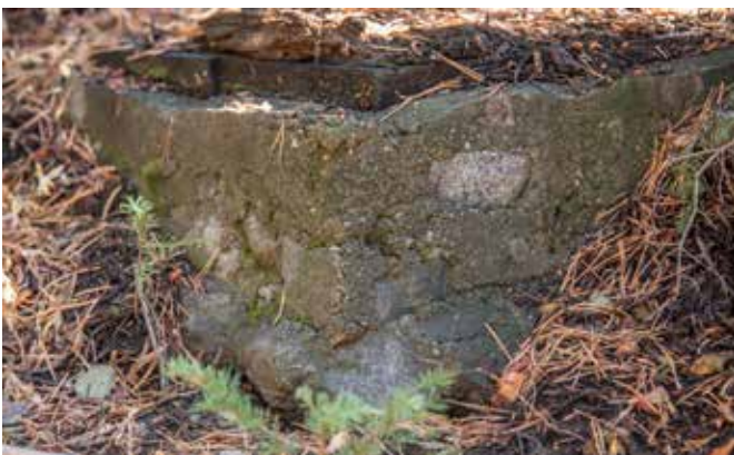
footing for the warming hut
