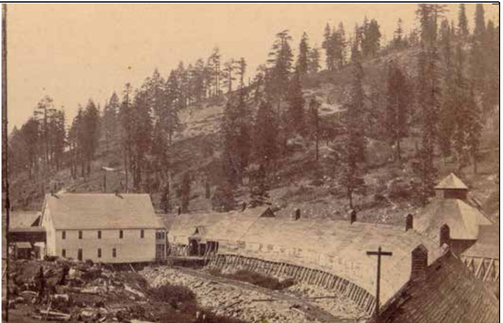
First Summit Hotel without its addition - about 1870. Structures to the right are the snowsheds leading to Tunnel 6. The building with the cupola is the roundhouse
