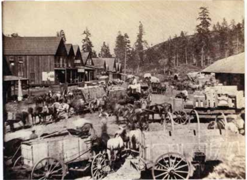
183. Main Street, Upper Cisco, 5,911 feet elevation.
