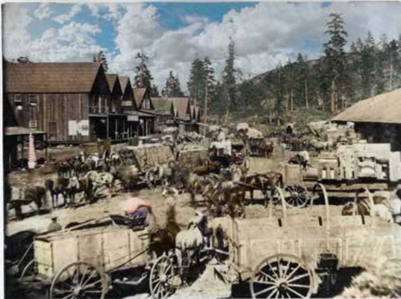
183. Main Street, Upper Cisco, 5,911 feet elevation.
