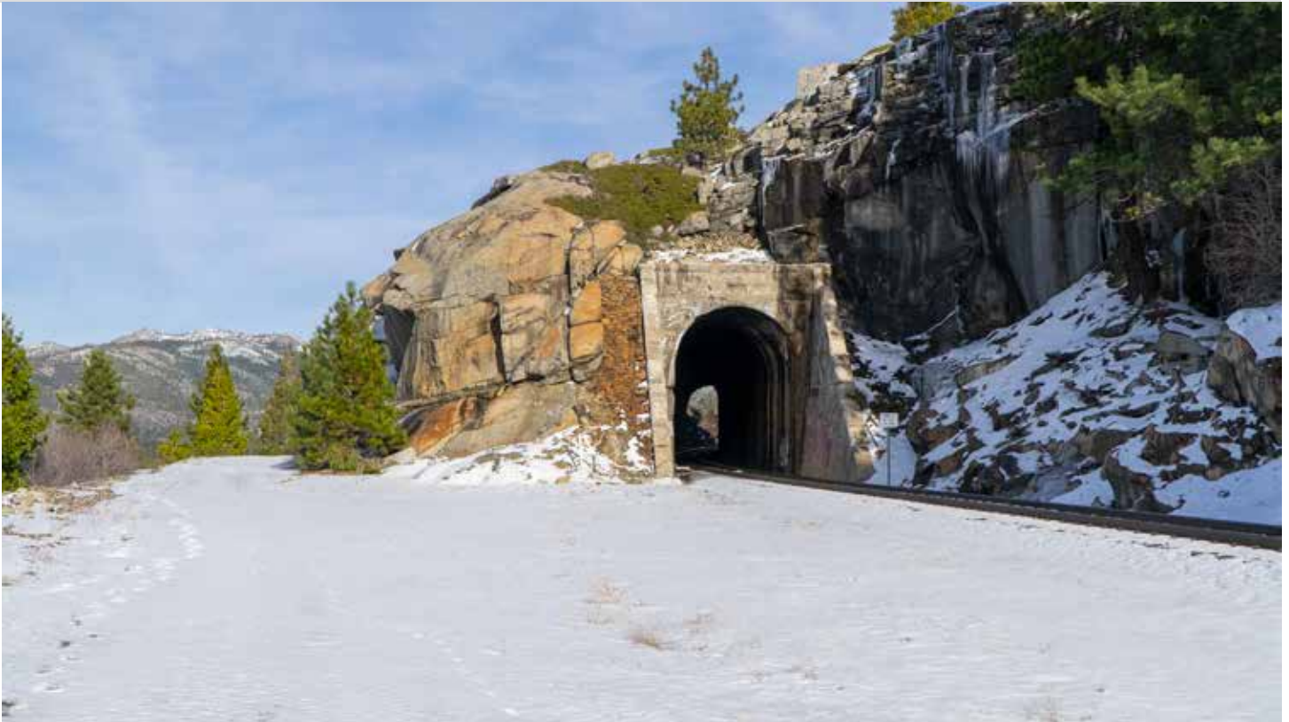
Tunnel 35 from 1924. This sits just above where Highway 20 joins I-80. It would be great to get a picture with Old Man Mountain and Red Mountain in the background but the geography just doesn't work.
