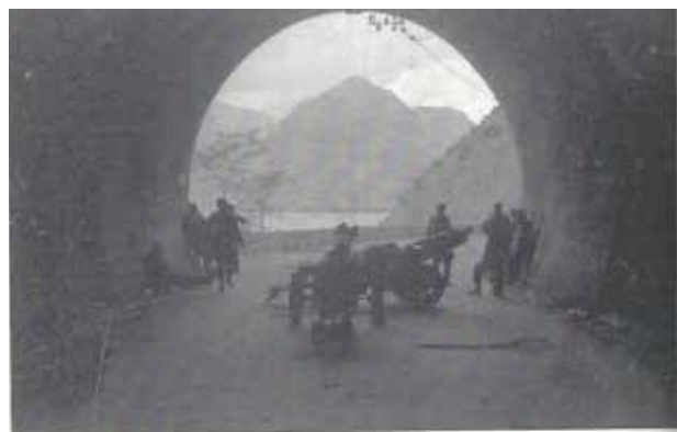
Highway tunnels on Lake Garda saw some of the last, grim fighting in northern Italy, late April 1945. (Richard A. Rucker)
