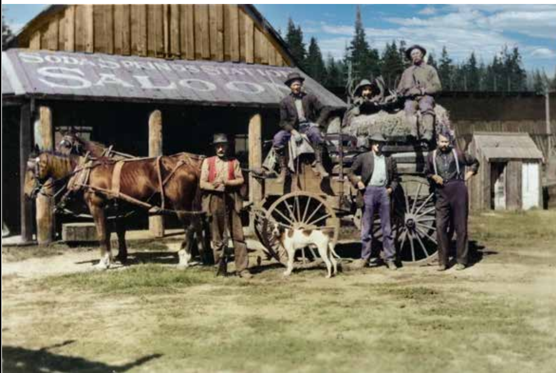
Soda Springs Station Saloon, today's Soda Springs, about 1900 which sat in what is now the parking lot for Soda Springs Ski Area. Note the snowsheds in the background that sat over forty miles of track. The view is looking north. You can see that Soda Springs Station was a thriving commercial hub.
