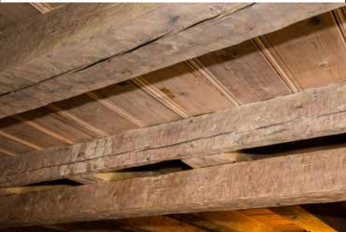
Rough hewn timbers in the ceiling of the basement.
