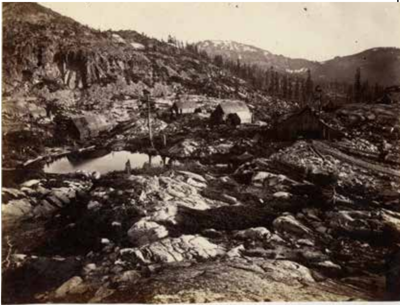
Alfred A. Hart #196 "Shaft House of Summit Tunnel ca. 1868. The building back, center, right, housed the donkey engine and the top of the central shaft of Tunnel 6. The pond is about where the Donner Summit Hub's parking lot is today.
